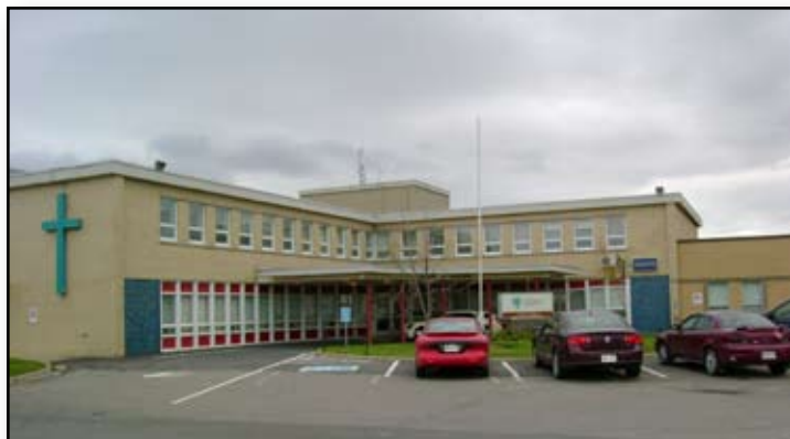
Lamèque Hospital and Community Health Centre
